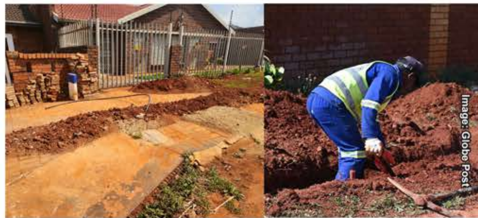
Workers continue with construction
