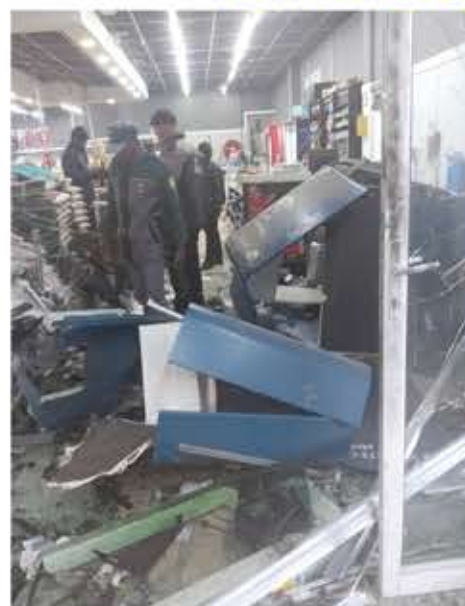
Visible damage at the store following the latest incident
