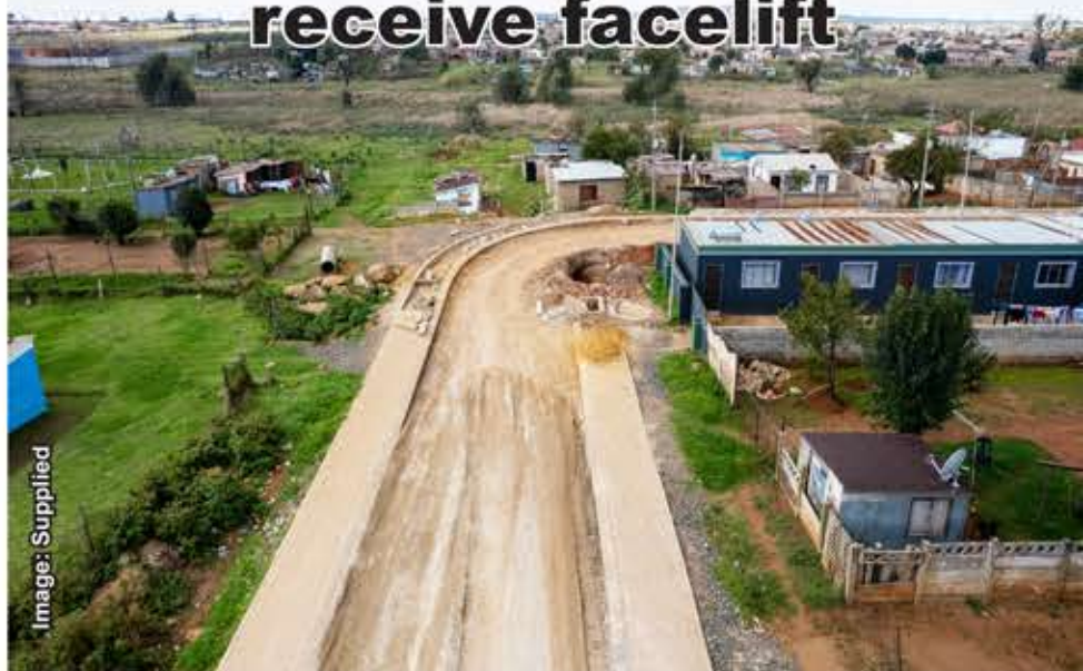
Construction underway to upgrade priority gravel roads
