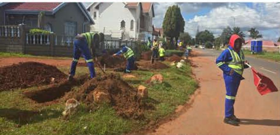
Installation in process on the corners of Sheffield and Lancaster roads
